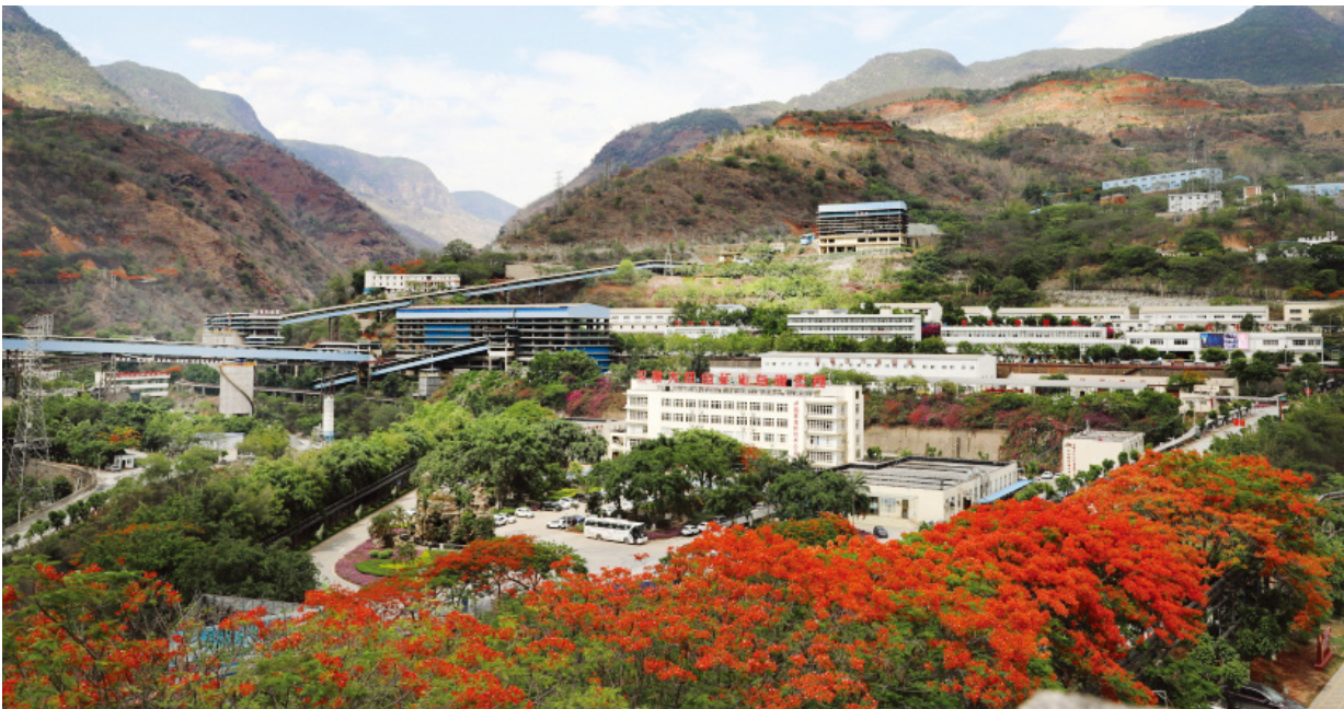
Construction of Dahongshan Mining tailings dam
